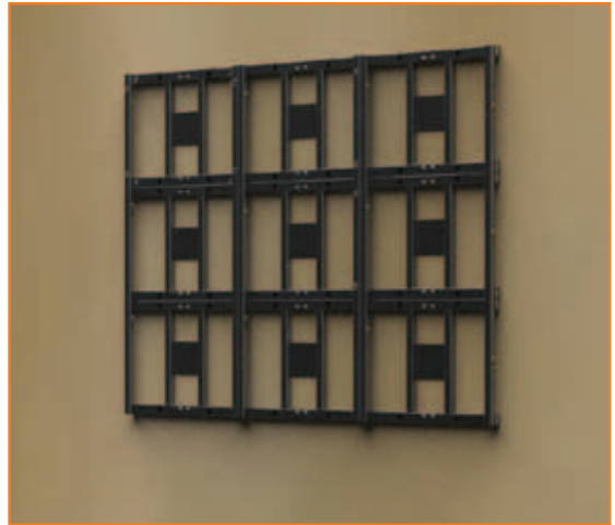
Install assembled frame work to a structural vertical surface.
